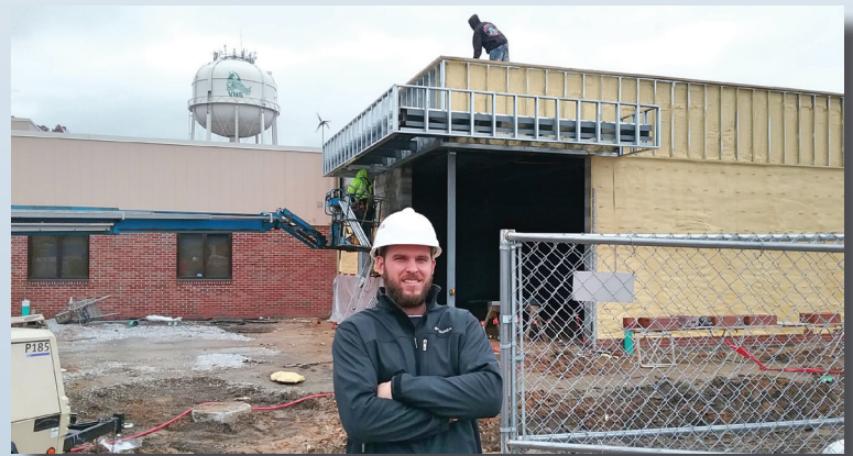
Site manager Will Hoefflicker oversees the Career Center renovation project.
